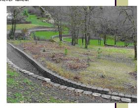
The lower loop required the least soil movement and once the excavator had completed a rough cut the bulldozer cleaned up the grade nicely. This is the upper side of the bottom loop, and the ground falls off very quickly to the left, out of picture, a short, low, level trestle is planned to span this gap. This was in October 2003.
