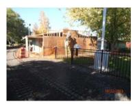
The fall weather gave us a break and we were able to get the building sealed before the rains could do any damage. Weather barrier was installed on the walls & roof and metal roofing was completed. The building was now weather tight.
