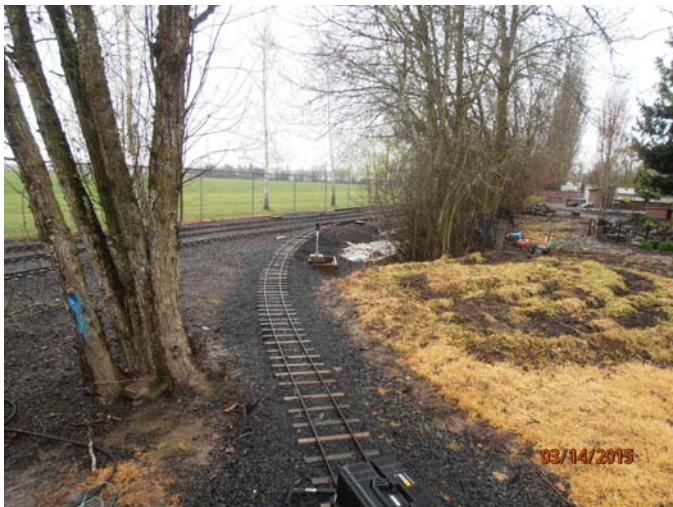
Signal from the industrial loop to the main line track.
