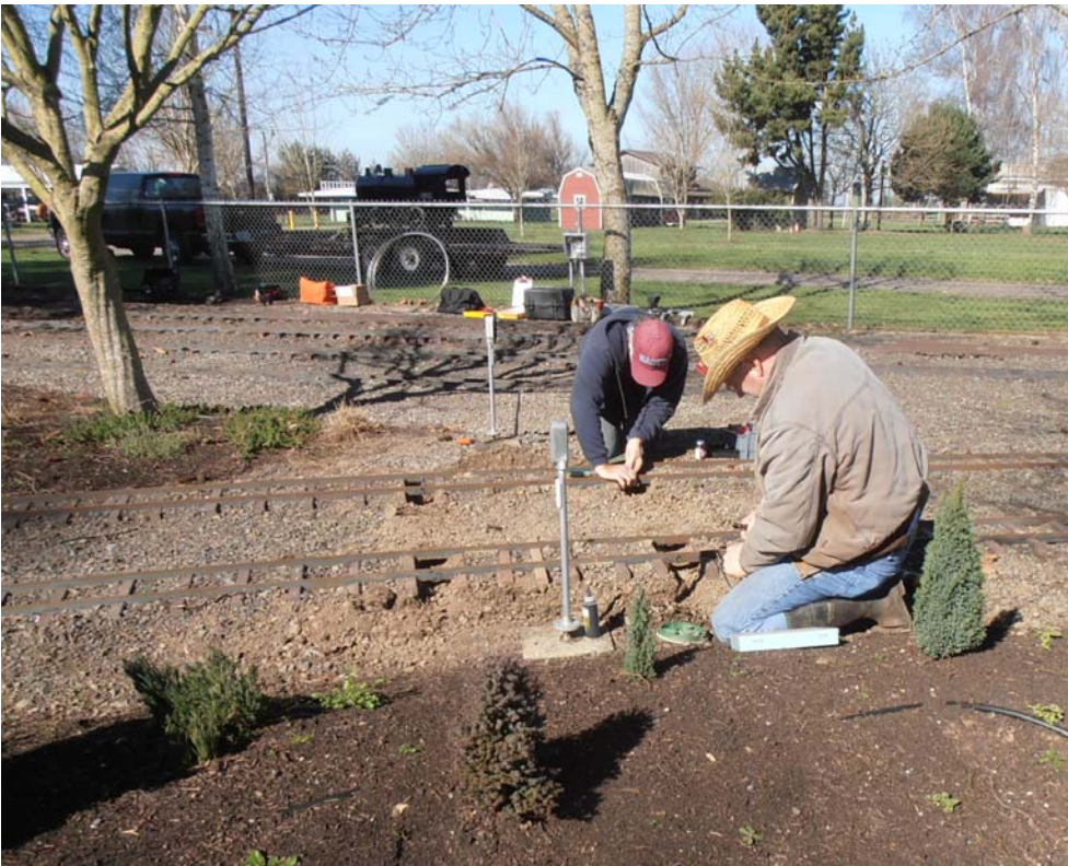
Blocks added for new signals.
