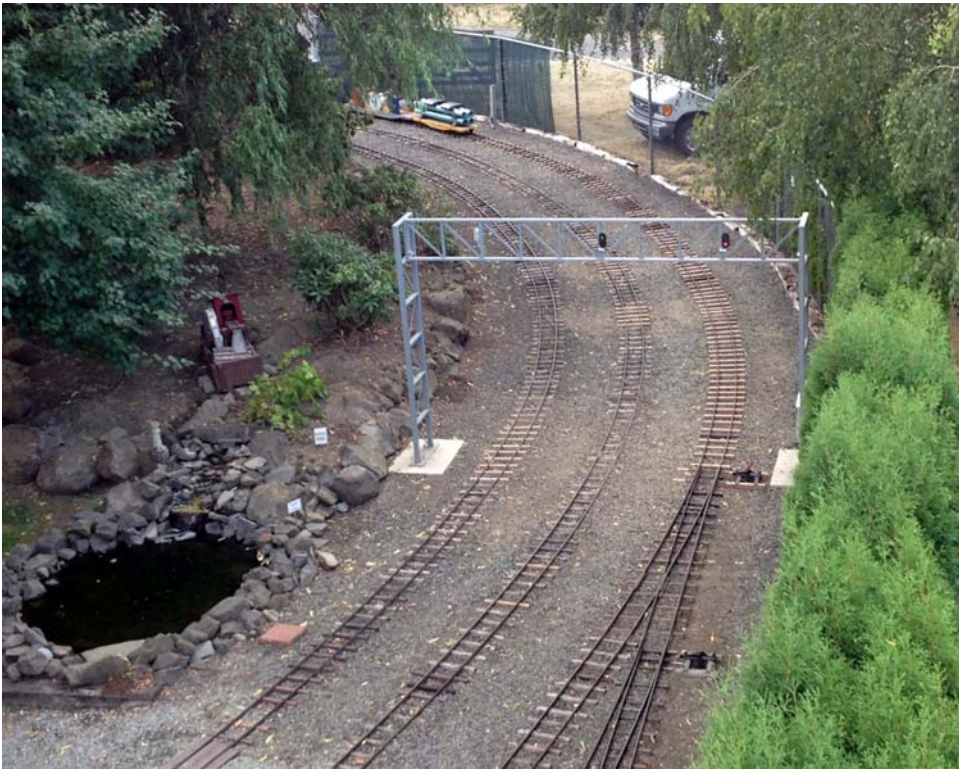
Signal bridge installed in 2013 allows control on the center track.
