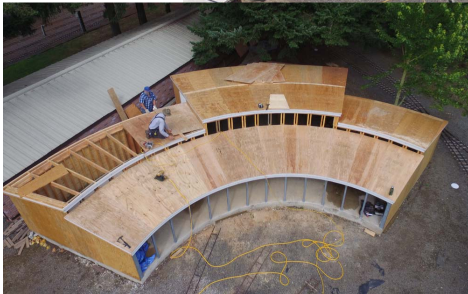
Roof sheathing almost completed.
