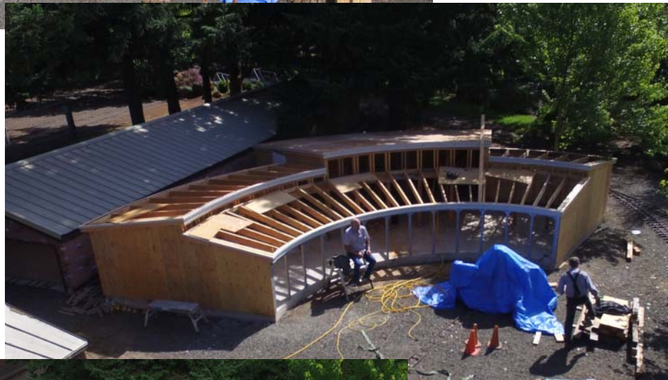
Walls completed and rafters installed. Starting roof sheathing.
