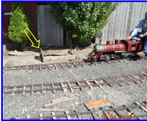
...signal bridge footing forms in place...
