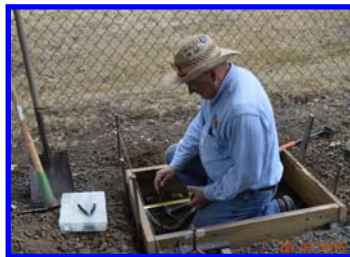
Alan installing electrical conduit for signal lights..
