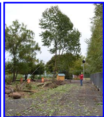
...second tree almost ready. (very windy)... A line was required to direct the fall.
