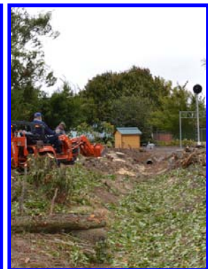
Wood removed. (1:30 pm)
