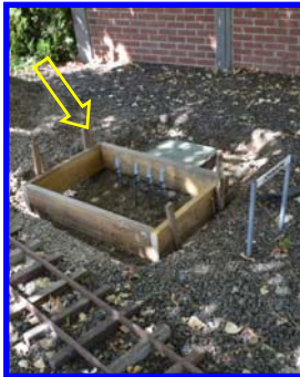
....ready for concrete.... (soon?)
