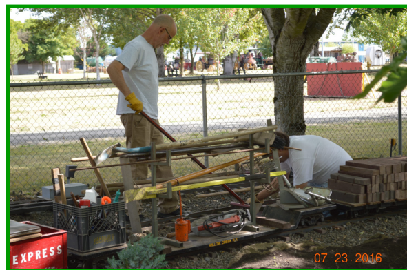
Pat & James replace northeast ties. East End Tie Replacement July
