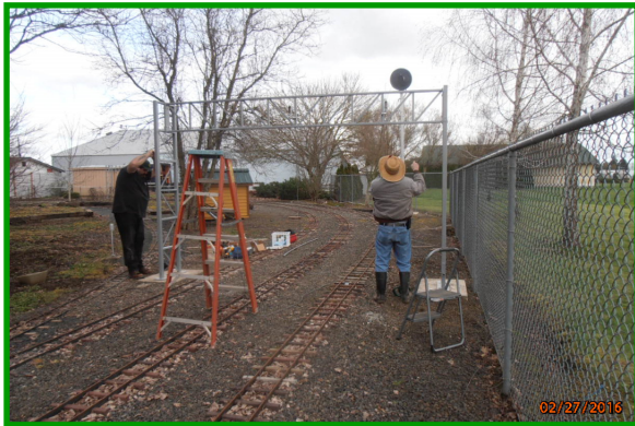
Noel & Alan pulling signal wires Southeast Signal Bridges Installed February
