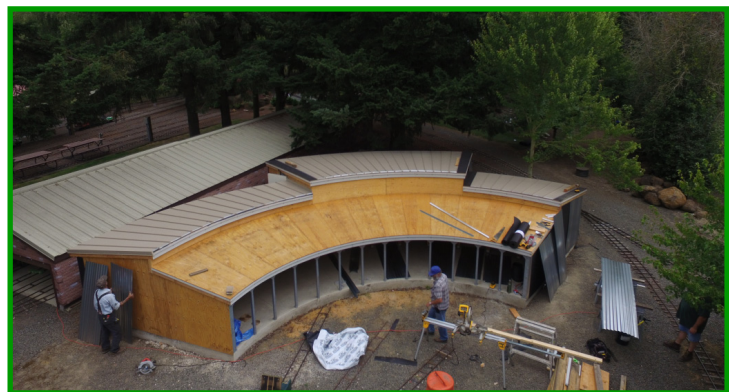
Phil L. & Vern install siding Roundhouse Progress July
