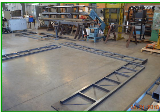
Metal cut for signal bridges. Welding ready to start. Chemeketa Students Start Signal Bridge Construction April -- June
