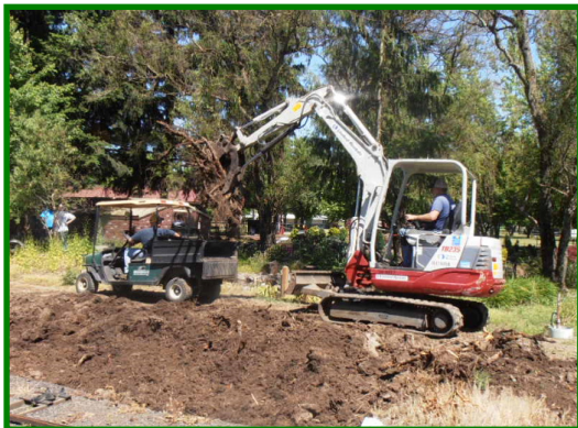
Evan removes remaining roots and prepares ditch for rock lining. Phil instructs members on proper excavation techniques.
