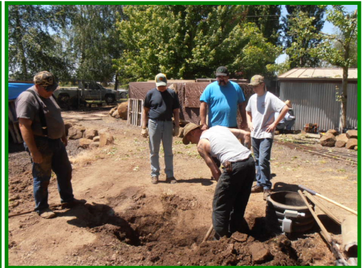
Evan removes remaining roots and prepares ditch for rock lining. Phil instructs members on proper excavation techniques.
