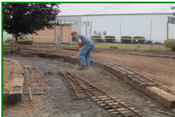
The previously placed Industrial-Loop track required re-alignment to allow placement of switch to the car barn track.
