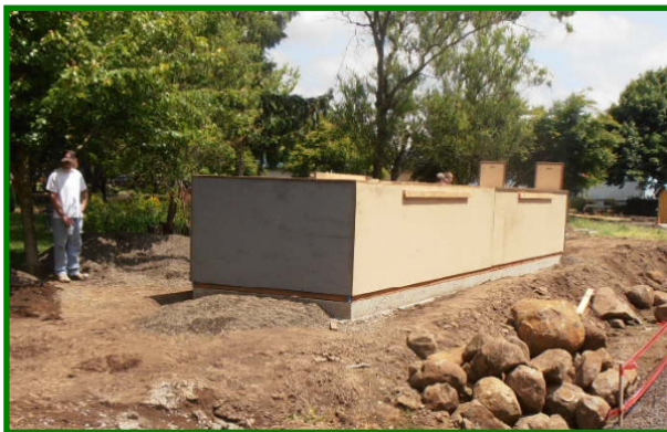
Both sections in place and waiting for a weather-proof roof and siding. At Alan's Kings Valley railroad, the car barn was set inside his pole building and did not require weatherproofing.
