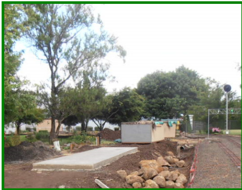
Steve Scharer poured a slab for the foundation. The first section is slid into place with the aid of Terry's tractor.
