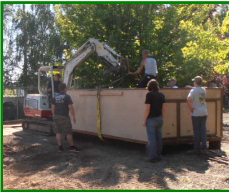
Car-Barn moves to unblock inner track loop before final placement. Note: Extra counterbalance required to keep excavator from tipping under load.
