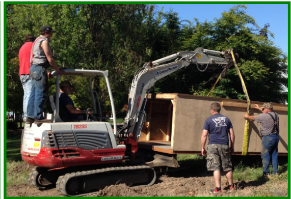
Car-Barn moves to unblock inner track loop before final placement. Note: Extra counterbalance required to keep excavator from tipping under load.
