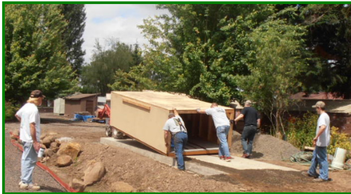
Steve Scharer poured a slab for the foundation. The first section is slid into place with the aid of Terry's tractor.
