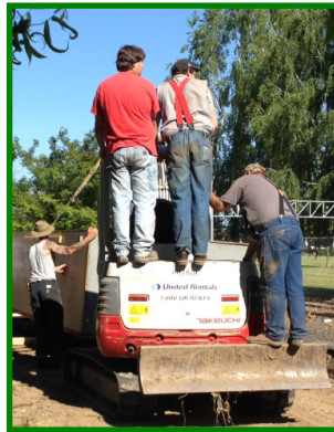
Car-Barn moves to unblock inner track loop before final placement. Note: Extra counterbalance required to keep excavator from tipping under load.
