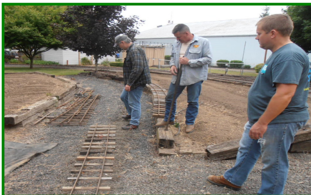
The previously placed Industrial-Loop track required re-alignment to allow placement of switch to the car barn track.
