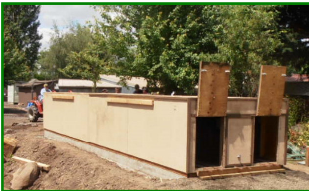
Both sections in place and waiting for a weather-proof roof and siding. At Alan's Kings Valley railroad, the car barn was set inside his pole building and did not require weatherproofing.
