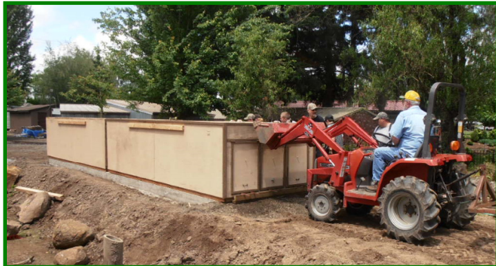
The second section is maneuvered onto the slab and nudged to mate to the first section.
