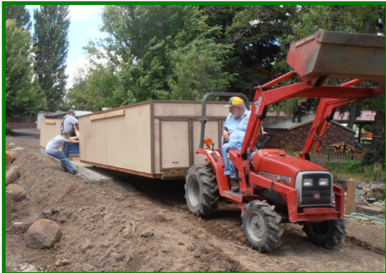
The second section is maneuvered onto the slab and nudged to mate to the first section.
