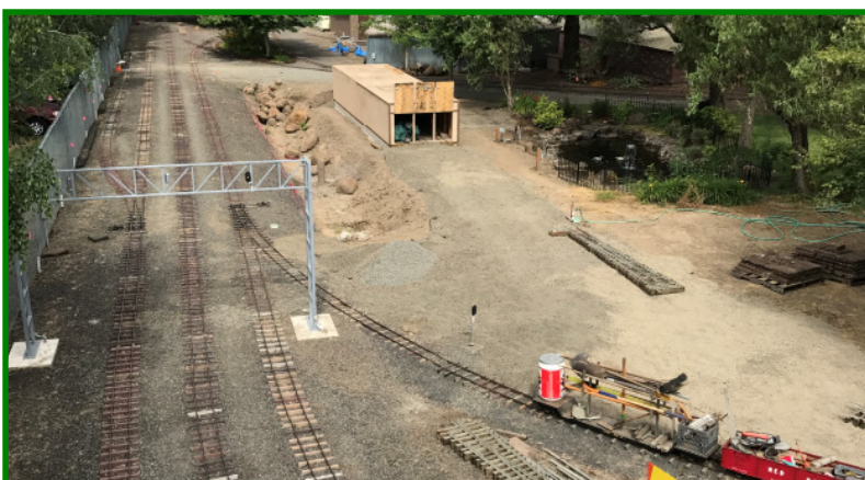
The previously placed Industrial-Loop track required re-alignment to allow placement of switch to the car barn track.
