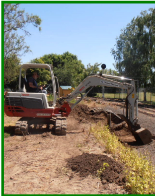
Evan removes remaining roots and prepares ditch for rock lining. Phil instructs members on proper excavation techniques.
