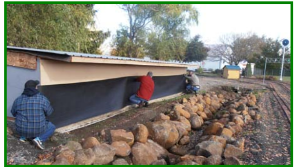
Scott, Mark & Alan apply building felt weather barrier
