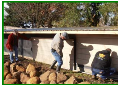
Mark, Alan & Frank apply temporary salvaged siding
