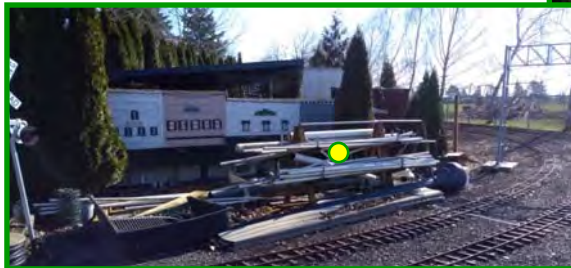
The ditch rock lining needs to be completed. The existing tracks next to the south side need to be lifted, tweaked and the ties refurbished.
