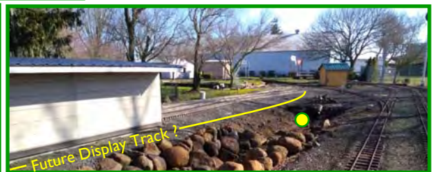
The ditch rock lining needs to be completed. The existing tracks next to the south side need to be lifted, tweaked and the ties refurbished.
