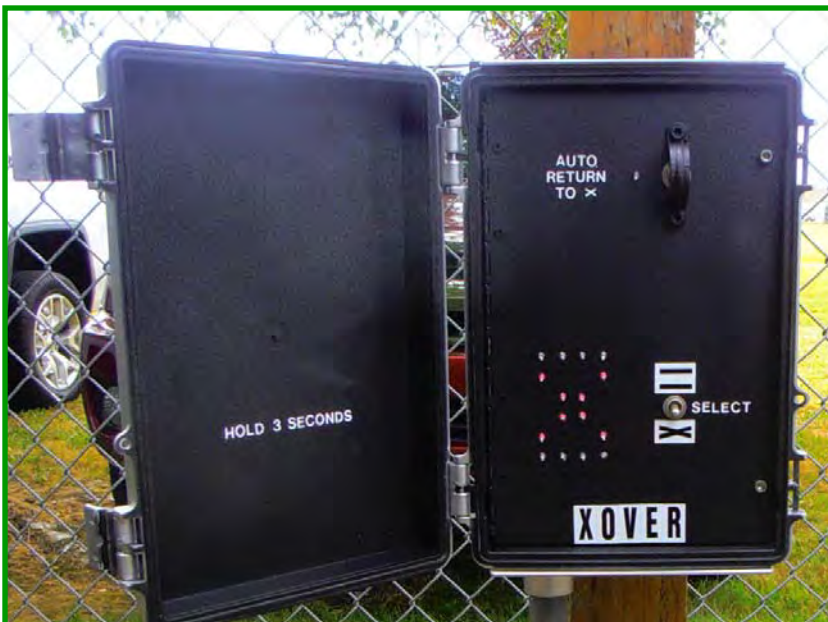
The "XOVER SELECT" switch must be held in the "||" or "X" position for three seconds to activate the electric switches. Both signals on the bridge go red until the switching process completes. This takes several seconds as each switch must turn individually in sequence.
