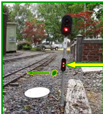
When this light is illuminated, the signal system is set in “Party Signal” mode.
