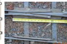
The turnout Frogs used at Willow Creek are machined from a single piece of steel.
