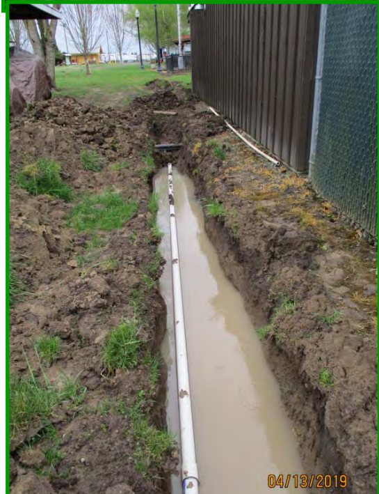
A portion of water supply has been connected to the new system. The ICP still needs to be connected to the existing water line inside the northwest storage room. The temporary wood floor in this area will have to be removed to accomplish this. The new water line would allow Willow Creek to have a year round water supply.
