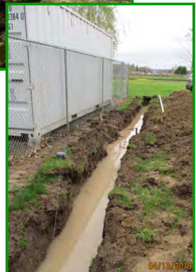
A portion of water supply has been connected to the new system. The ICP still needs to be connected to the existing water line inside the northwest storage room. The temporary wood floor in this area will have to be removed to accomplish this. The new water line would allow Willow Creek to have a year round water supply.
