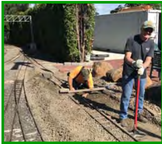
Ernie & Dave prepare grade for new ICP train platform.
