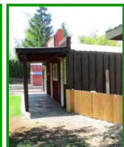
The completed fence.
