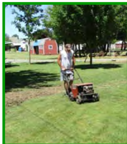
The lawn on the east side of the ICP is prepared for seeding. This area was disturbed by the new water line construction. Roy tills the area where the cottonwood tree was removed years ago. Garry aerates the lawn with the plug cutter. Mark uses the tractor to back-drag the area where leveling dirt was placed. Trevor uses the screen roller to tamp the grass seed into the soil.
