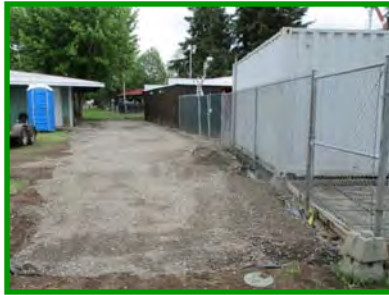
The new gravelled area north of the ICP. This should help to reduce the wet weather mud at the north entry gate.
