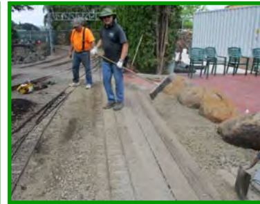
Gravel is placed at the platform.
