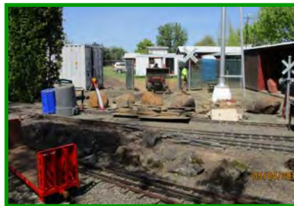
The last of the gravel leveling course is being placed.
