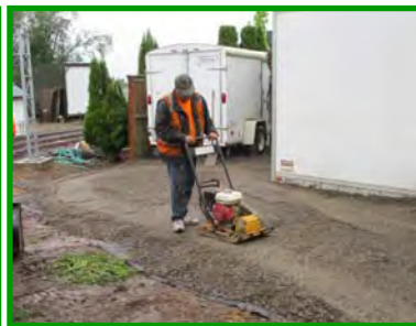
The tree stumps have been removed behind the Nelson container. Ernie compacts the new gravel pad so the pipe storage racks may be returned to their former location.
