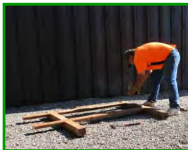
Support members added to posts.
