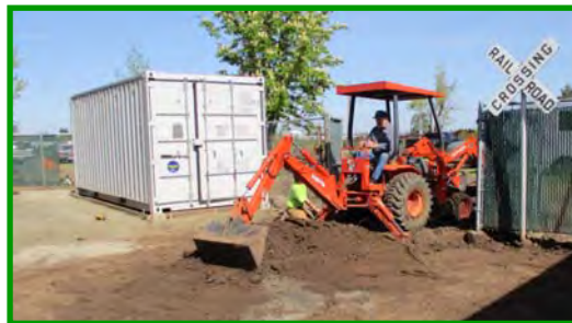
Steve completes grading behind the ICP.
