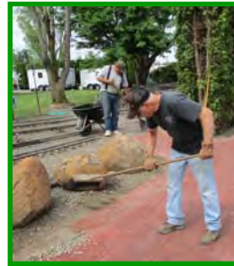
Dave and Ernie finish dressing the new slab edges with gravel.
