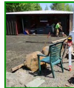
The leveling gravel has been watered down and compacted.
