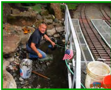
Frank performs the unpleasant task of removing accumulated muck from the waterfall pool.
