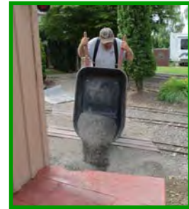
Dave and Ernie finish dressing the new slab edges with gravel.
