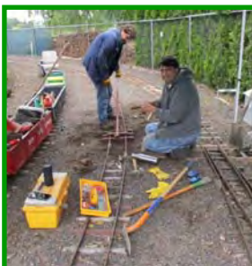
Jesse & James replace deteriorated main line ties.
