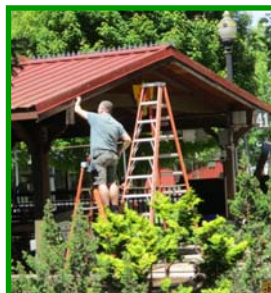
Darin Installs Flashing
