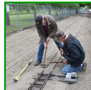
Track Panels Lined
