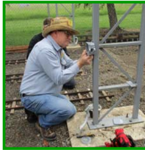
Alan Installs Turnout Control
