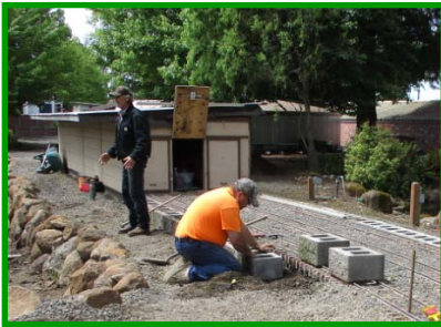
Ernie Places Retaining Wall Block
