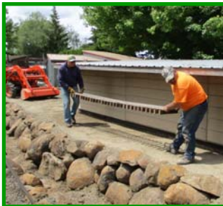
Track Panels Located
