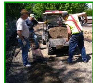
Jeff & Nate Place Ballast
