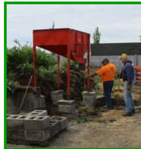
Ernie Places Gravel Bunker
