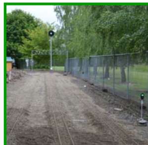
Track Panels Ballasted
