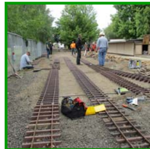
Track Panels Placed
