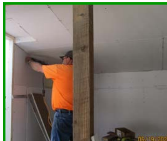
June 19 th : Sheetrock nearing completion
