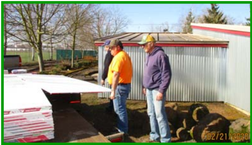
Feb. 21 st : Sheetrock & Supplies Delivered.
