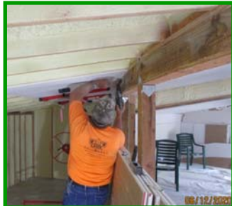
June 12 th : More Sheetrock
