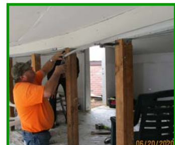
June 20 th : Corner Trim Installed.
