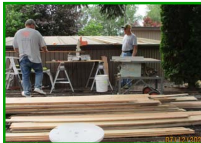
July 12 th : Trim Boards for Posts and Windows
