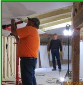
June 5 th : Continued Sheetrock
