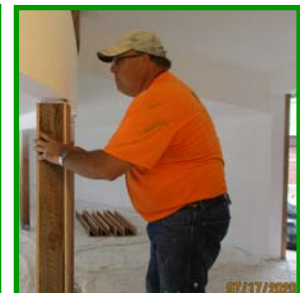
July 17 th : Post Covers Completed
