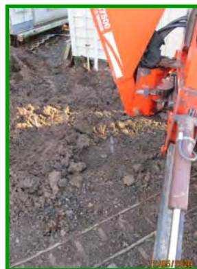
Ernie carefully backfills the new trench. Unfortunately some of the existing conduits were very close to the surface requiring extra care.
