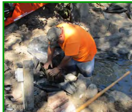
A sand base and perimeter wall blocks have been installed. The new liner is positioned for placement. Rock is added around the perimeter as the liner is adjusted.
