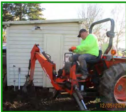
Ernie carefully backfills the new trench. Unfortunately some of the existing conduits were very close to the surface requiring extra care.
