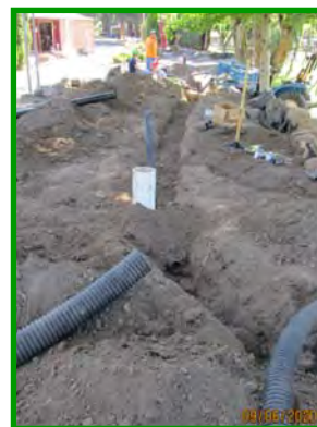
Backfill is compacted behind the perimeter rock. Coyote Ridge has been expanded and conduit placed for the new water feature and other items.
