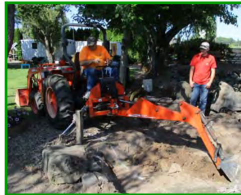
The old pond liner and gravel is removed. The tractor is used to enlarge the pond.
