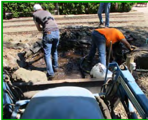
The old pond liner and gravel is removed. The tractor is used to enlarge the pond.
