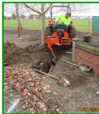
Rumley assists Ernie with placement of the tractor. Finally a conduit is placed under the track. The water line is placed through the conduit to connect to the existing water line on the south side.
