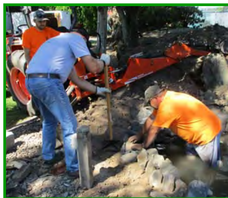
Backfill is compacted behind the perimeter rock. Coyote Ridge has been expanded and conduit placed for the new water feature and other items.
