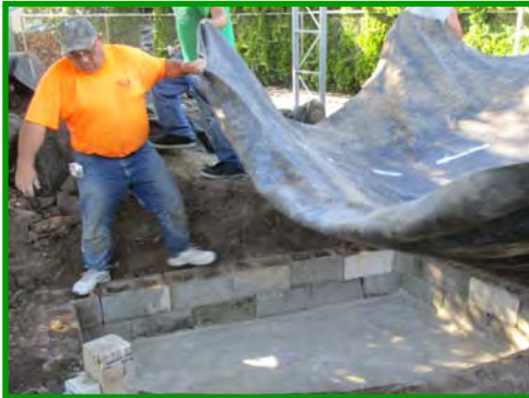
A sand base and perimeter wall blocks have been installed. The new liner is positioned for placement. Rock is added around the perimeter as the liner is adjusted.
