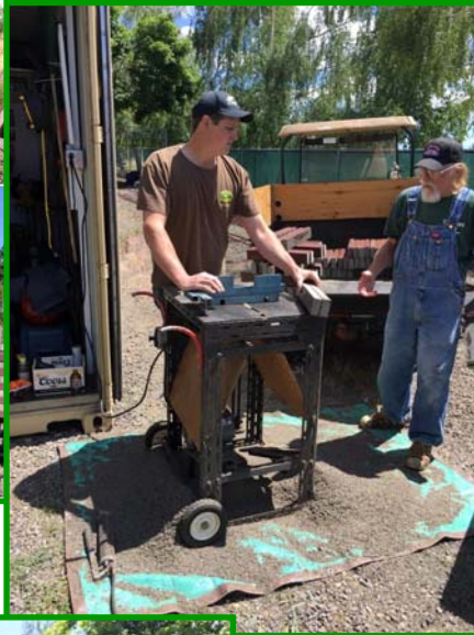
Second step in tie replacement. Notch the ties by Nate and Garry. (First Step: Cut the trex boards to length and width by Evan and Dave @ Evan's shop)
