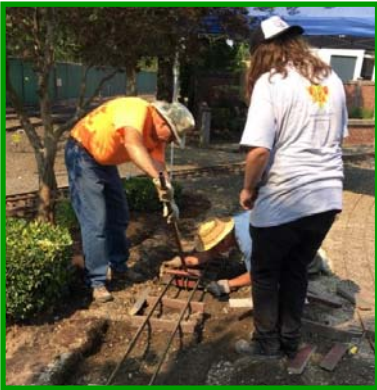
This section of track had ties from the original rebuild. Treated with used motor oil, they did survive for many years
