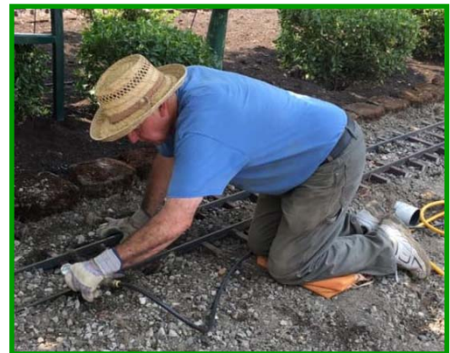
A conduit is installed for future utilities. Ballast is tamped using compressed air.
