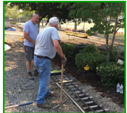
This section of track had ties from the original rebuild. Treated with used motor oil, they did survive for many years
