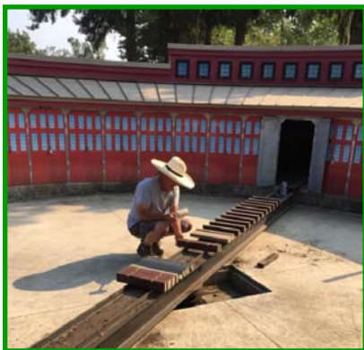
The new track jig is used to install ties. The finished product! Ready for more years of service.
