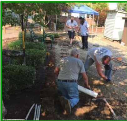
A conduit is installed for future utilities. Ballast is tamped using compressed air.
