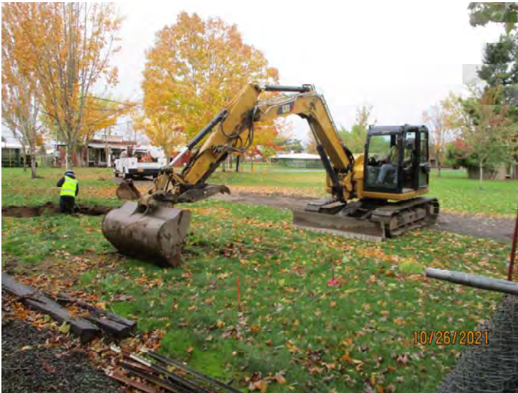
The footing excavation was donated by Willamette Valley Excavating.
