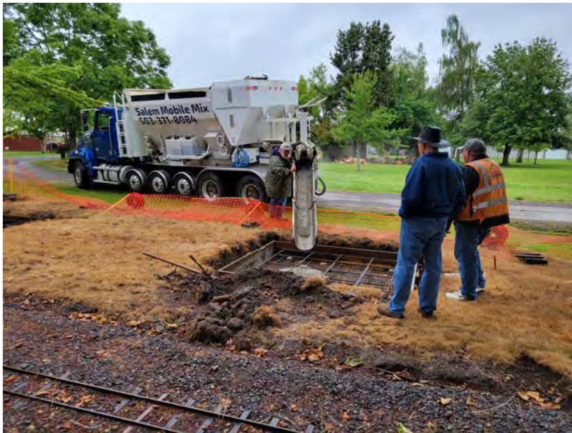
Concrete for the footings was installed.
