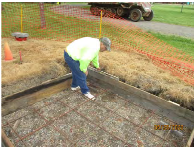
Formwork was completed and checked. Reinforcing steel bars were installed.
